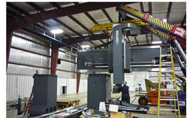
50 ton twinlift setting a machine
