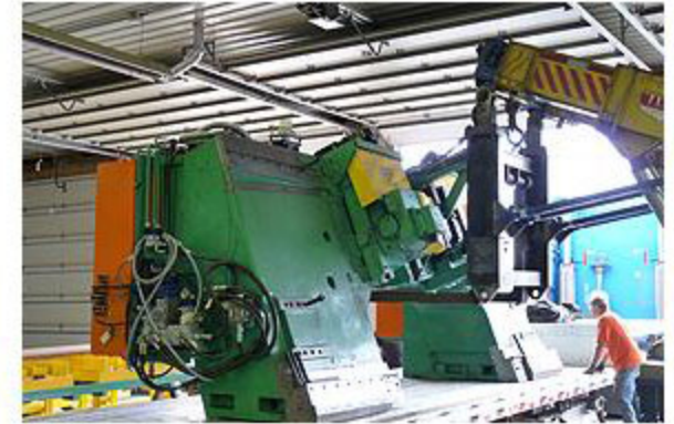
34 ton twinlift with fork attachment unloading a machine sitting flat on truck floor
