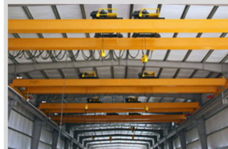
Bridge and jib crane installation and inspections
