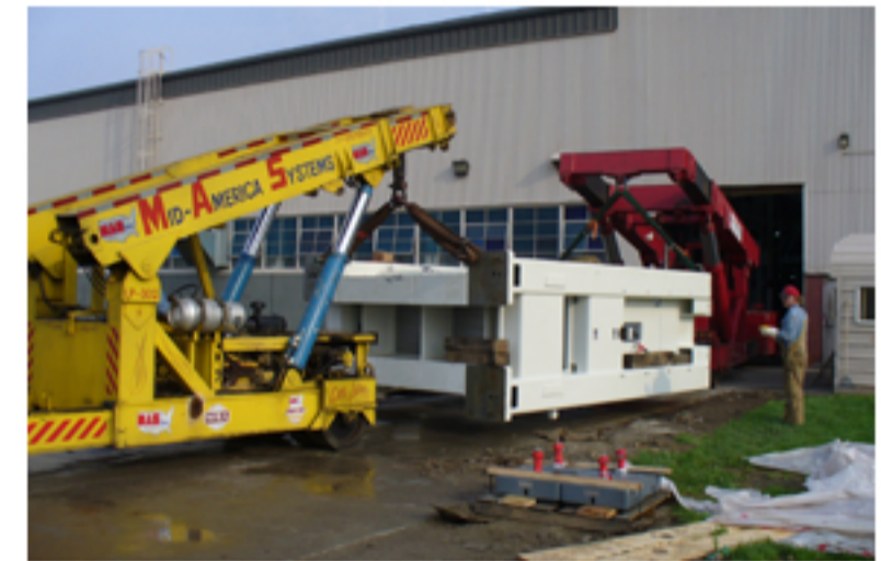
Two twinlifts at work installing a press in low head room facility
