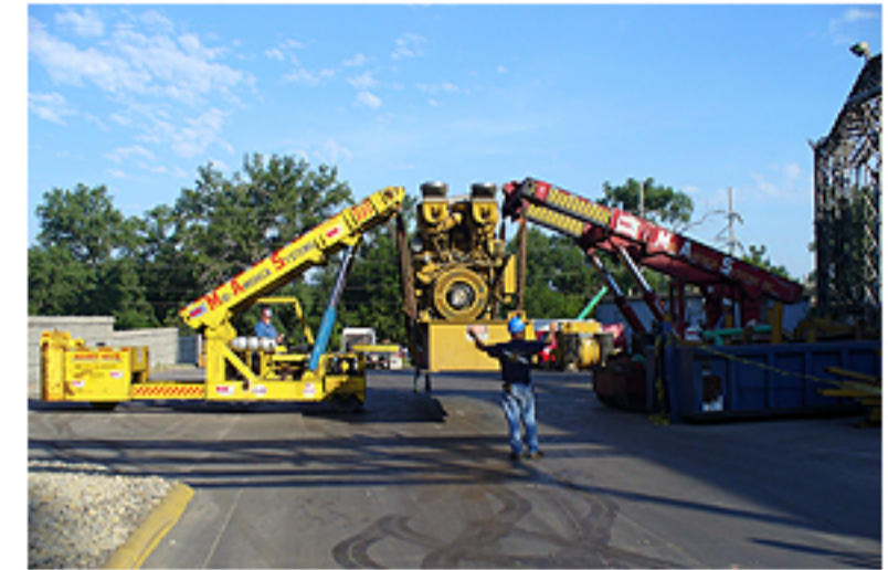
2 twinlifts lifting a gen set onto a truck
